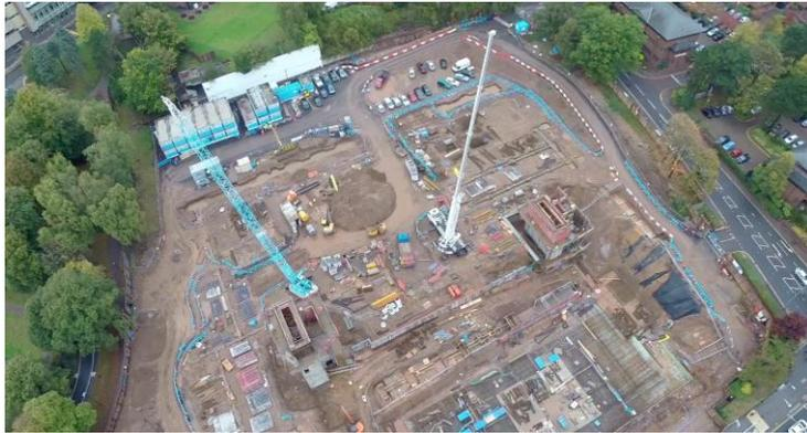
Following completion of the bulk excavation works, substructure (foundation) works have progressed well, and are now complete to the “Central Building” and Pool Hall area; foundation works to the Sports Hall are currently progressing well.
